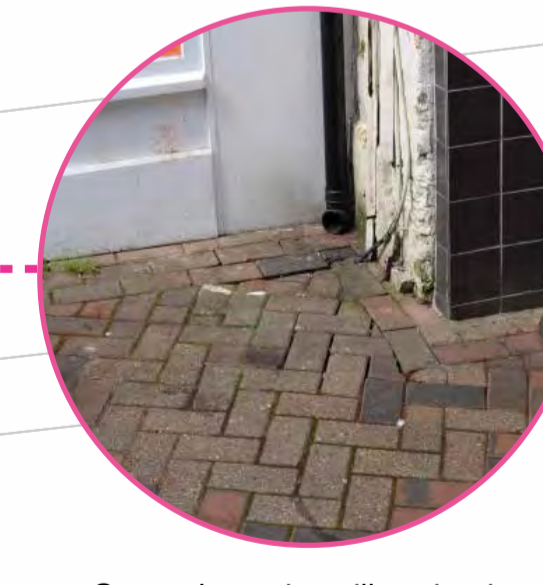
Some downpipes ill-maintained causing rain water to discharge down the sides of the building Looks scruffy and creates negative impression
